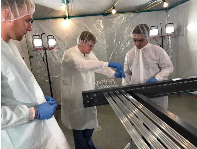
*Figure 2: Construction of the sub-module zero of the field cage for the qualification of the FRP I-beams production companies.*
