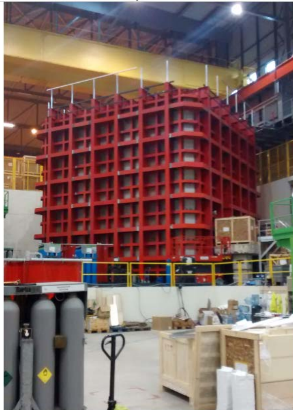
Fig.5: Completion of ProtoDUNE-DP cryostat exoskeleton assembly.
